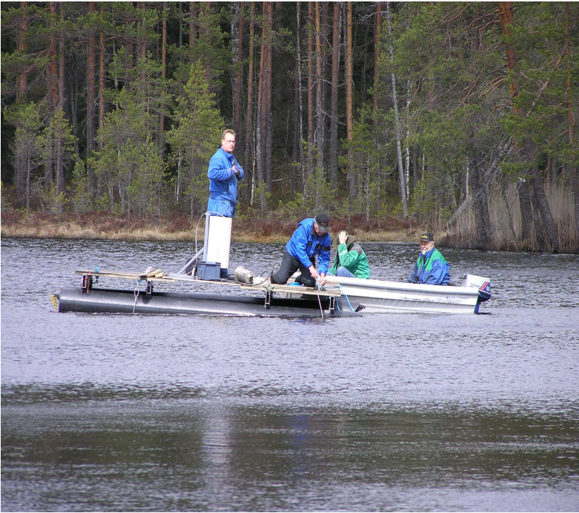
Figure 3. Installation of the mixing equipment (MIXOX) in lake Halsjärvi, May 4 th 2005.
